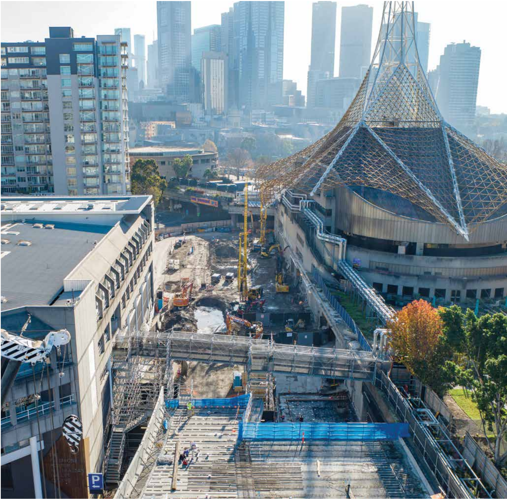
An aerial view of MAPT works behind Arts Centre Melbourne.
